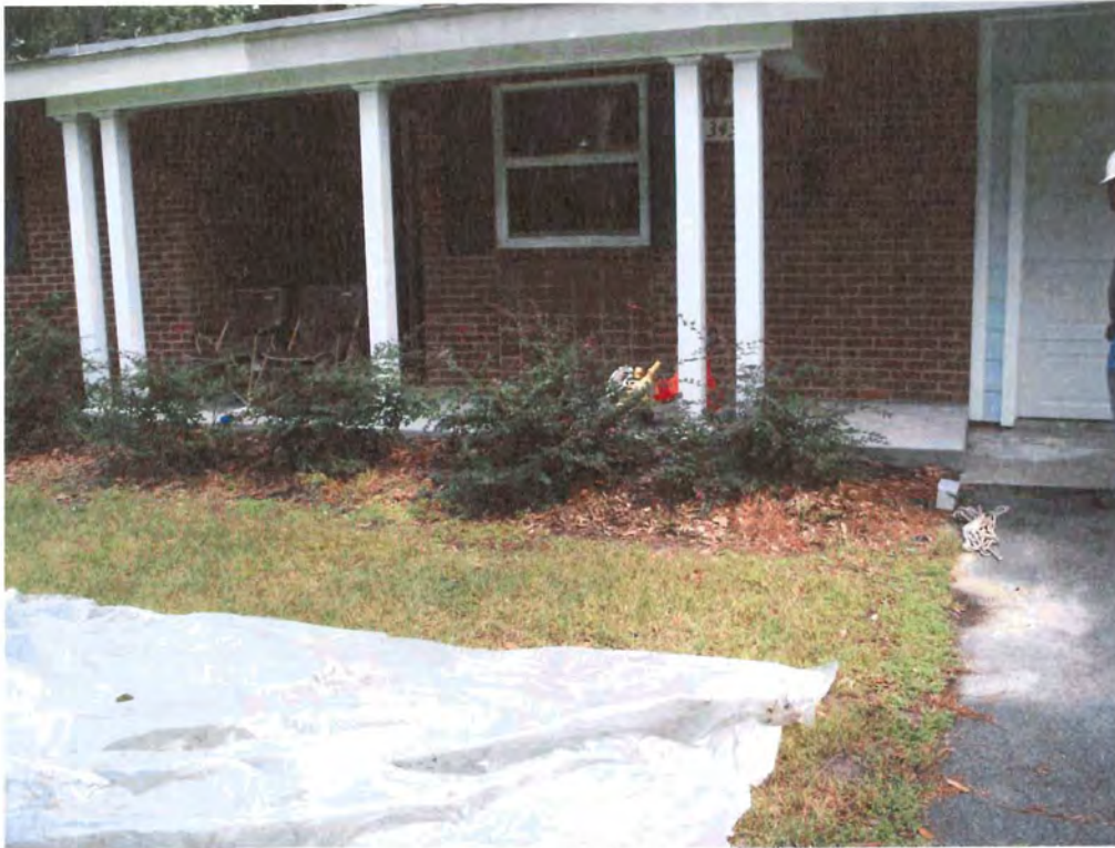
Picture 1: Location of UST 343Ash-1 and 343Ash-2.
